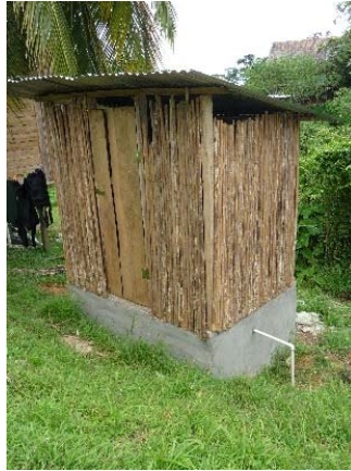
Figure 9. Double-Vault Urine-Diversion Composting Latrine in a Ngäbe Community in Bocas del Toro Province (Courtesy of Author)
